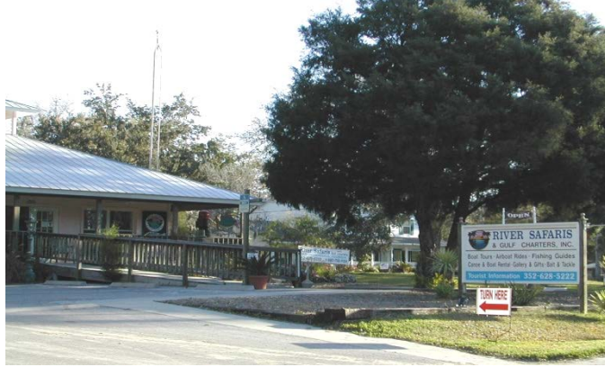
Nonresidential Stemwall Construction
